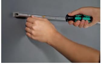
Screw the plastic profile to the wall  $\dots$
